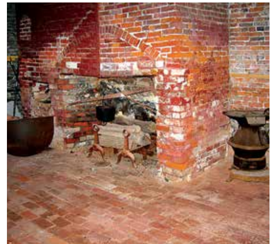
Below: Open hearth fireplace and bake oven in the Back Kitchen—our next renovation project.
